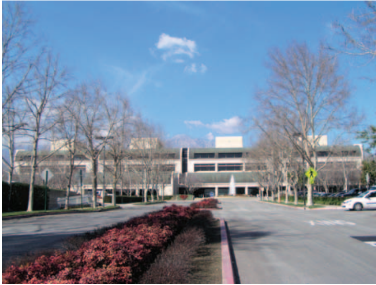
Figure 8. Foothill Communities Law and Justice Center, Rancho Cucamonga, California—First Base-Isolated Building in the United States
