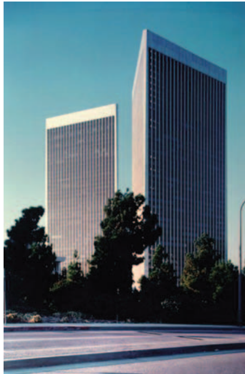
Figure 3. Century City Theme Towers, West Los Angeles
